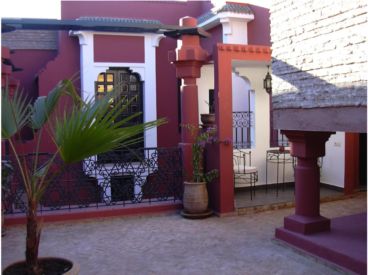
Detail of multi tiered roof terrace; consists of many intimate nooks.
